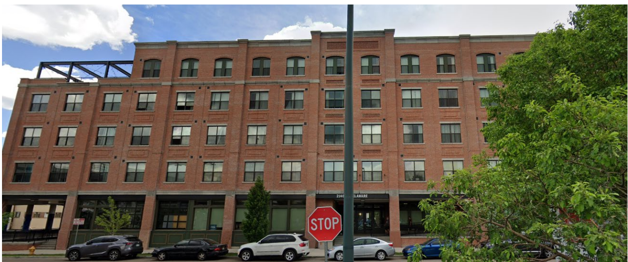
West – from Delaware St. Source: Google Maps
