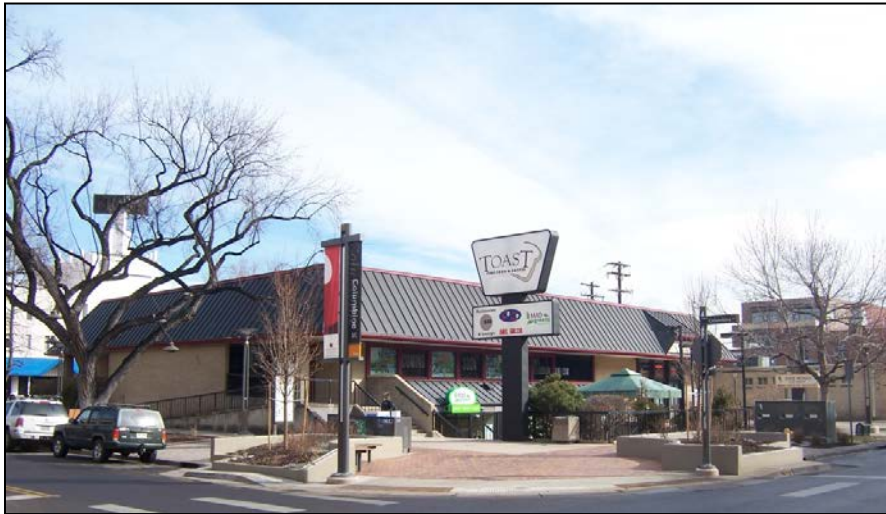
200 Columbine Street, viewed from the corner of 2 nd & Columbine looking northeast.
