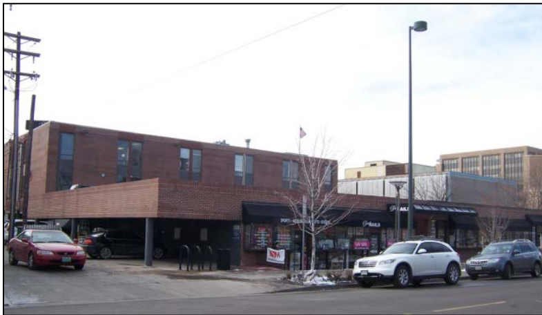
The 3 rd Avenue frontage of 2600 E. 3 rd Avenue, viewed from the intersection of 3 rd Avenue and the alley between Columbine and Clayton Streets, looking southwest.
