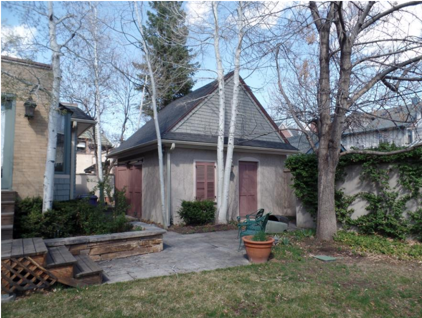
Carriage house from the south
