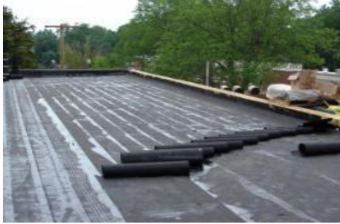
Built-up Roof (BUR)
