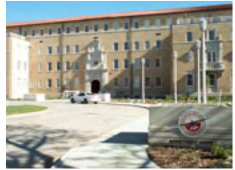
The Grand Lowry Lofts is a mixed-income project that required a combination of public and private financing.
