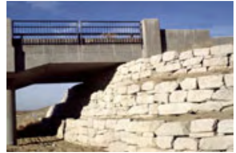
Infrastructure construction at the Stapleton site.
