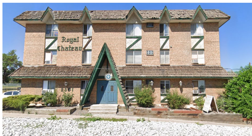
East of subject property, facing west from South Federal Boulevard
