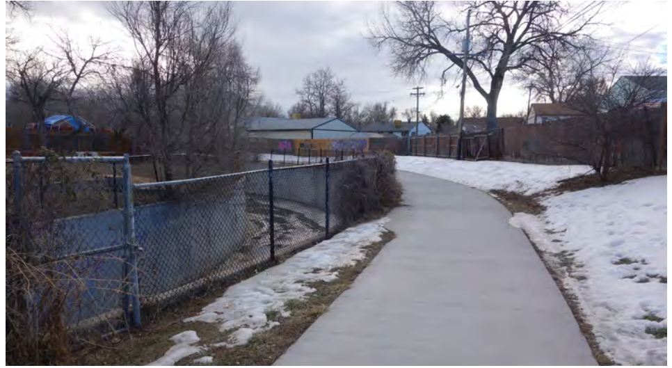
WEIR GULCH: EXISTING CONDITION
