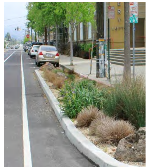
Bump-out Stormwater Planter
