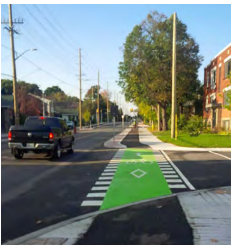
Intersection Crossing Markings- Ottawa, CA
