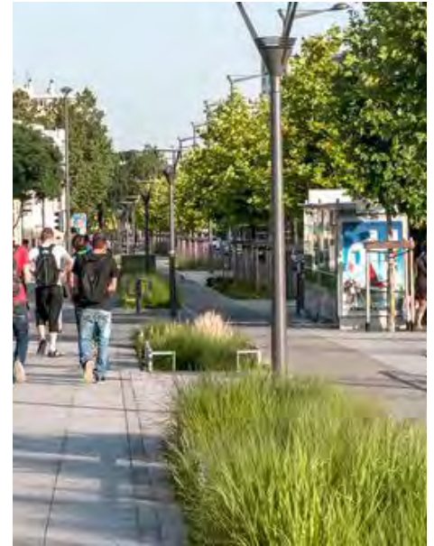
Streetside Stormwater Planter
