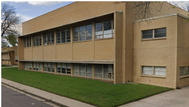
Two-story church use west of the subject site, facing east from S. Grove Street
