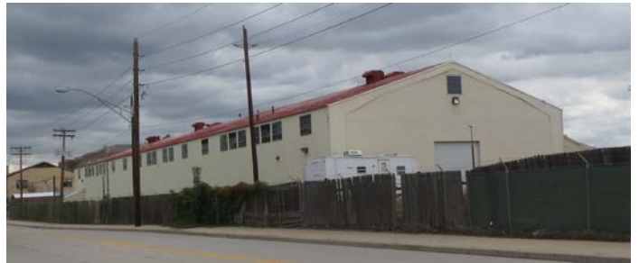
5- Buckley Annex non-residential structure, 2 story, directly east of subject property
