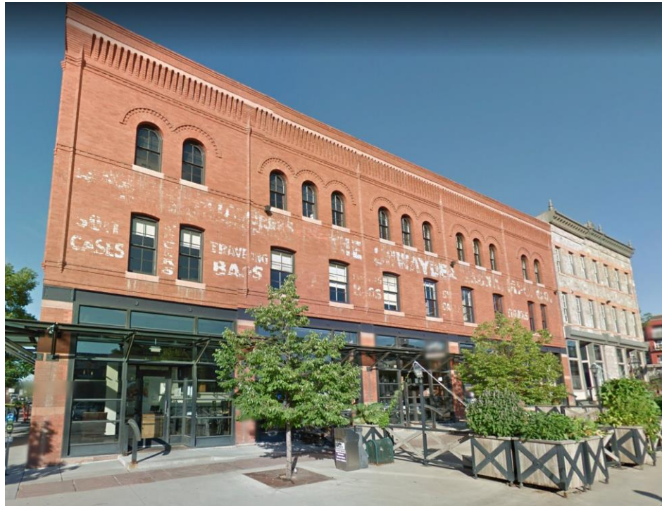
1553 Platte Street – Former Shwayder Trunk Mfg. Co. factory
