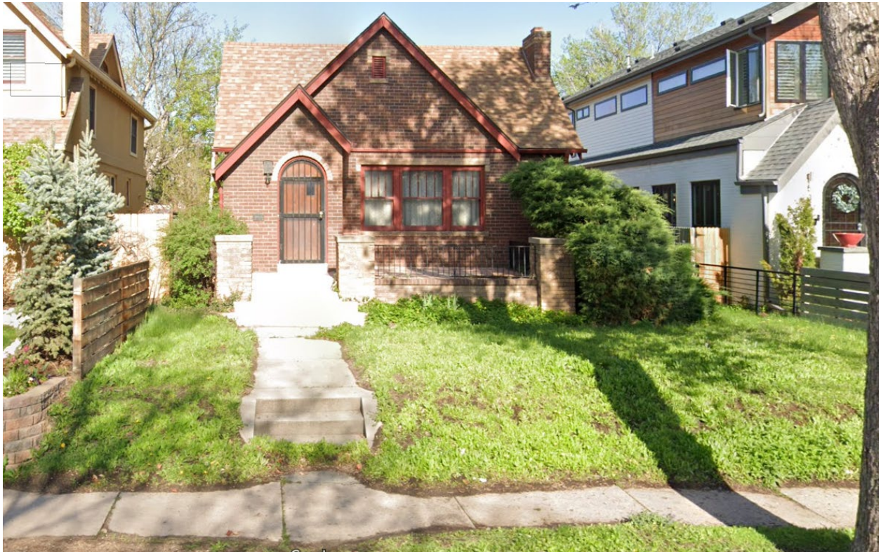
View of the property to the south, facing east (Source: Google Maps)
