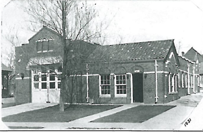
Fire Station #3, c. 1931. Courtesy of Denver Public Library, Western History Department, C Photo Album 111. Denver Fire Department
