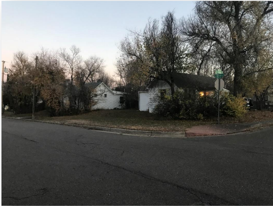
Figure 1: 1188 Quince St. (Two Small Houses on a Single Lot)
