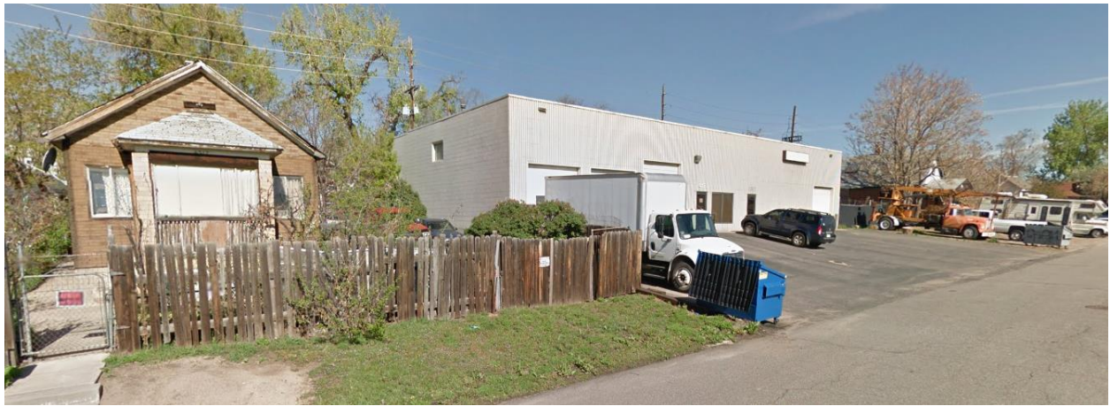
One-story, single family residential structure and one-story industrial building to the south of the subject site, looking north
