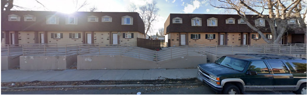
Subject Site (1409-71 North Julian Street) - View of the subject property, looking West (on North Julian Street)
