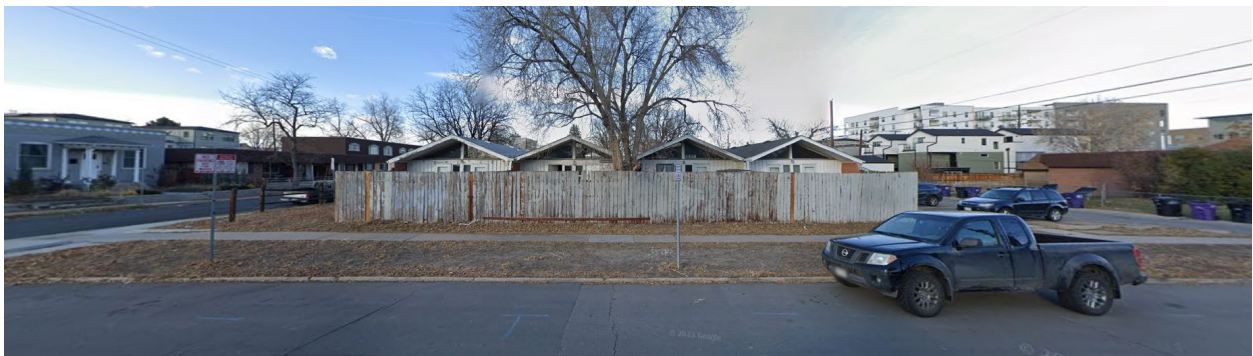
West - View of properties to the West of West 14 th Avenue, looking North (on West 14 th Avenue)
