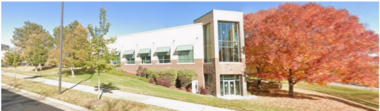
View of the remaining property to the west from East Belleview Avenue looking north
