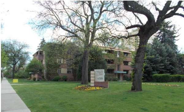
Photo looking southwest from Downing Street at Country Club Gardens
