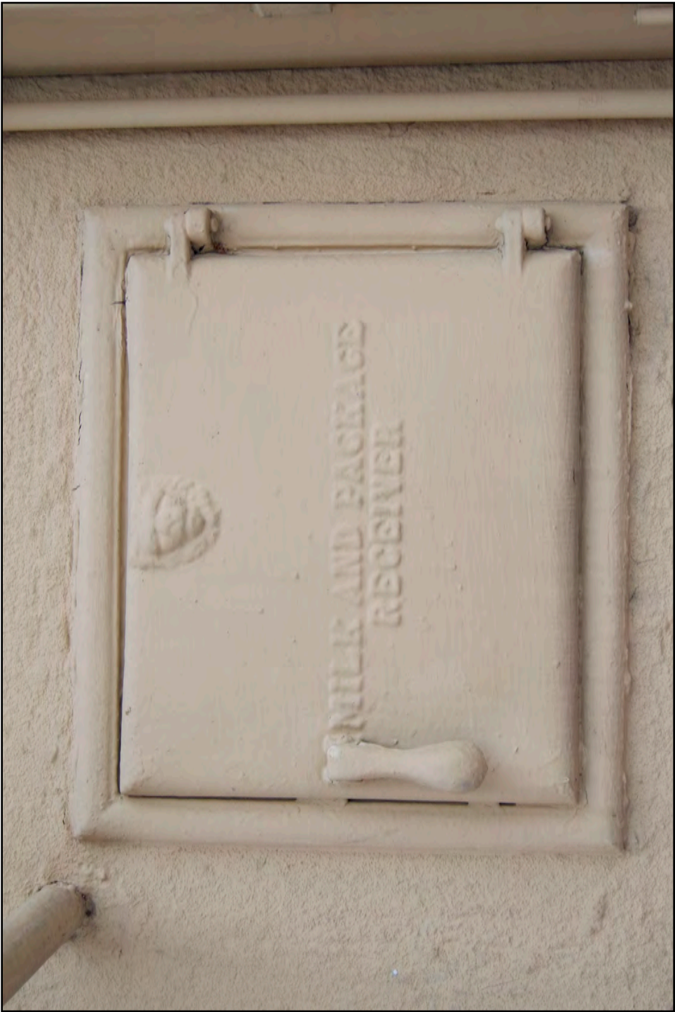
Door for milk and package delivery on the rear of 119 E. Vassar Ave.
