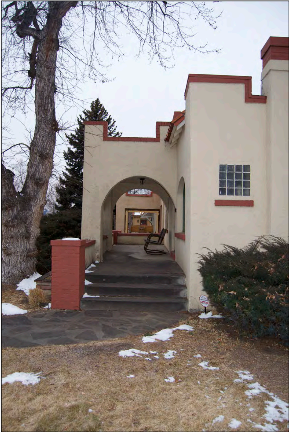
Looking west from 119 E. Vassar Ave. to illustrate line of sight between porches
