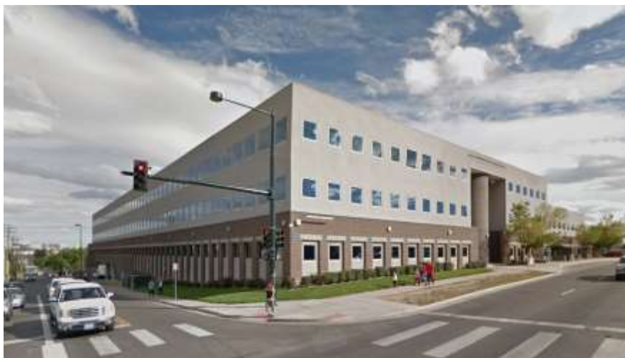
View of Denver Human Services building, west of the subject site, looking east from Holden Place and Federal Blvd (Source: Google maps)
