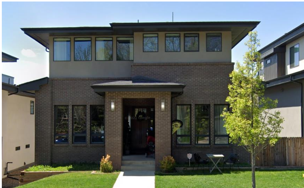
View of the subject property, facing west.
