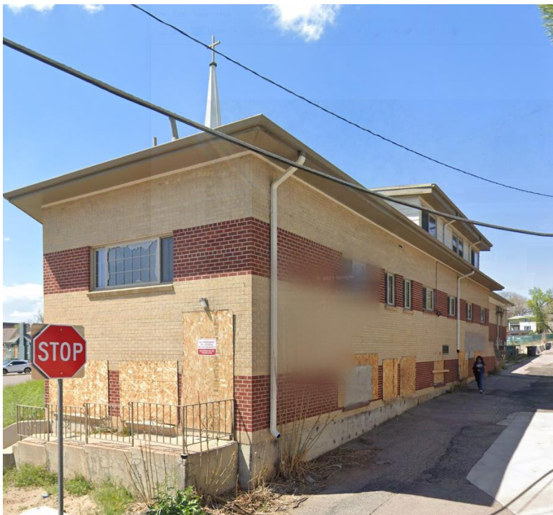
View of the property to the west, behind subject property and alley, facing northwest.
