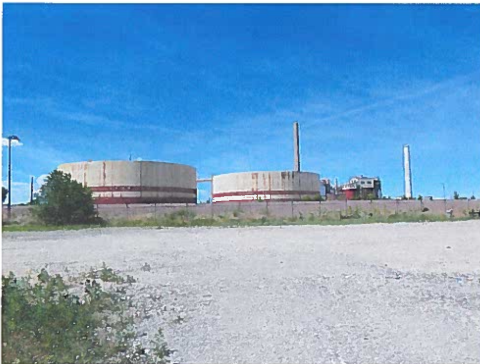
Vacant lots along West 11th Avenue in front of the defunct tank farm and Zuni Station
