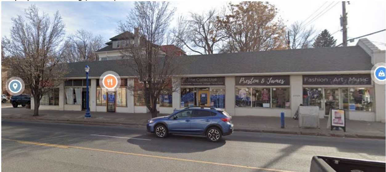
View facing south on E. Colfax Ave. between Milwaukee and Paul St. in the Congress Park neighborhood – within proposed rezoning (U-MS-3)
