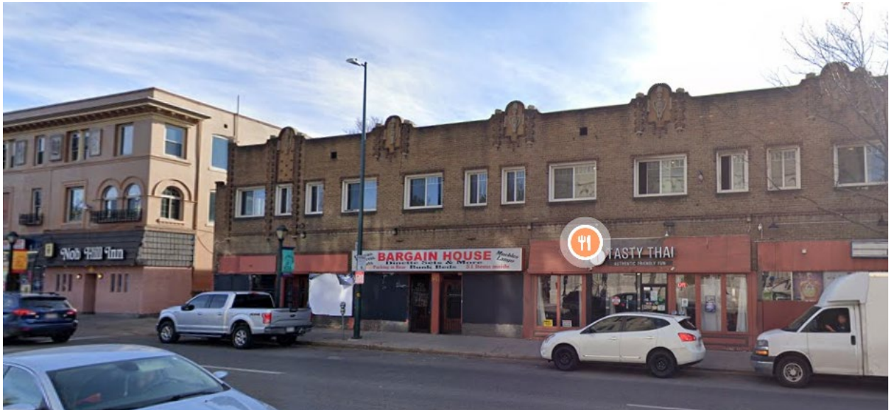
View facing south along E. Colfax Ave. N. Grant and N. Logan St. in the Capitol Hill neighborhood – within the proposed rezoning (C-MS-8)
