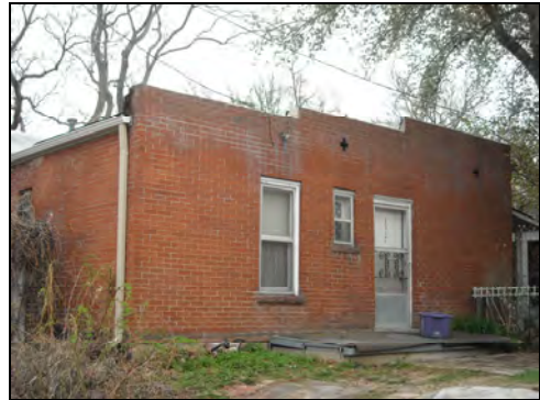
Secondary house, 3317 W. 29 th Avenue
