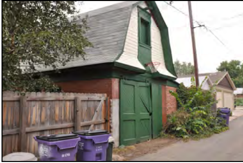
Barn/garage, 3405 W. Hayward Place
