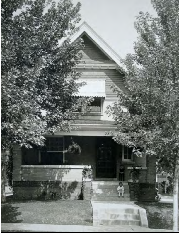
Figure 14. Charles J. Starke erected the house at 3395 West 30 th Avenue in 1909. SOURCE: Jane and James Hinkle, Denver, Colorado.
