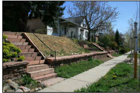
Stone retaining walls/steps, W. 29 th Avenue
