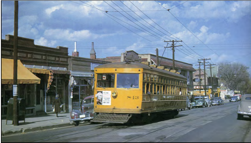
Figure 17. The West 32 nd Avenue business district north of the district was a busy neighborhood shopping area in 1950, the year streetcar lines to the area were abandoned. SOURCE: Richard H. Kindig photograph, 13 May 1950, view east-northeast of the 3600 block, in Robertson, et al, Denver's Street Railways, 1901-1950 , vol. 2 (2004), 520.
