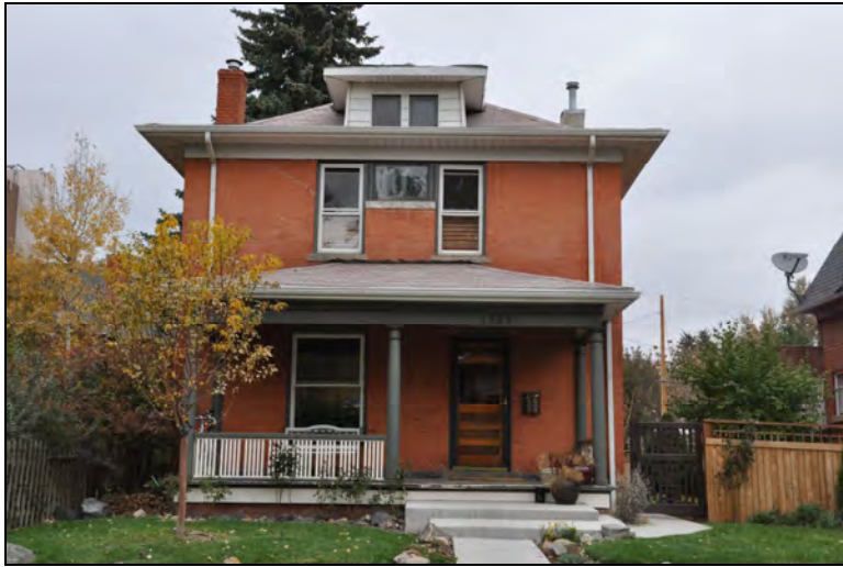
Boyles House (1903), 3383 West 31 st Avenue
