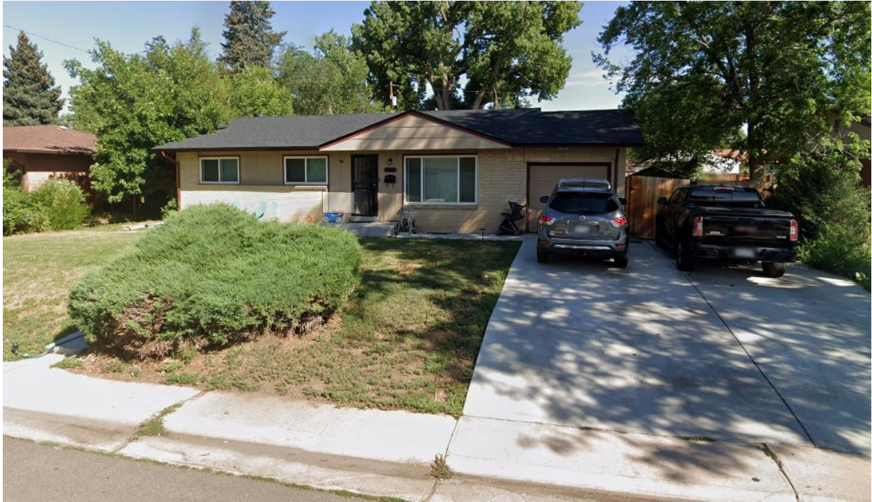
View of 3443 S Patton Way, looking north. (Source: Google Maps)
