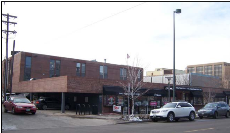
The 3 rd Avenue frontage of 2600 E. 3 rd Avenue, viewed from the intersection of 3 rd Avenue and the alley between Columbine and Clayton Streets, looking southwest.
