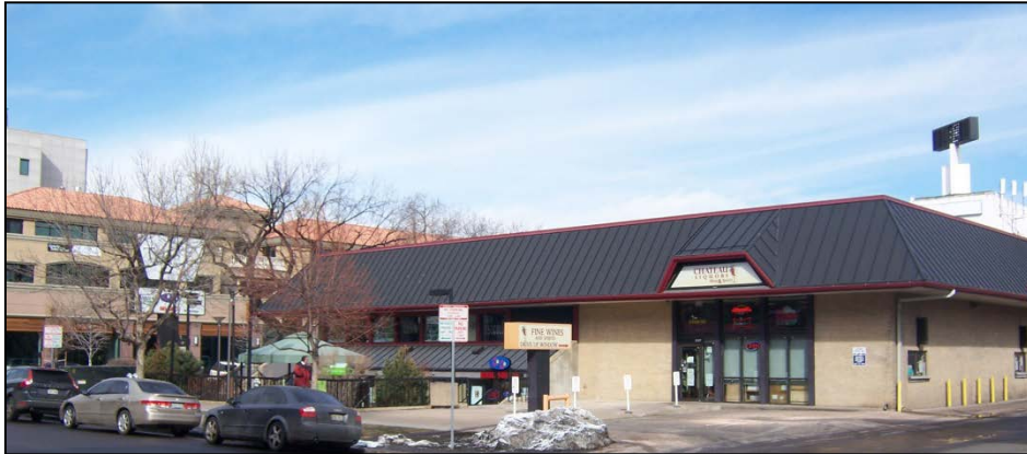
The 2 nd Avenue frontage of 200 Columbine Street, from the corner of 2 nd Avenue & the alley between Columbine and Clayton Streets, looking northwest.
