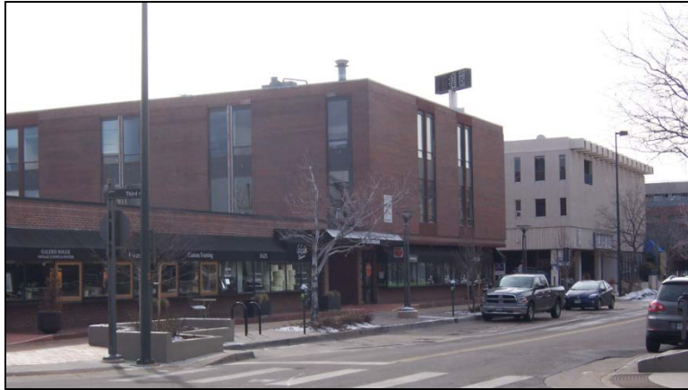
2600 E. 3 rd Avenue, viewed from the intersection of 3 rd Avenue and Columbine Street, looking south-southeast.
