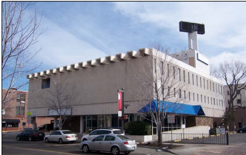
234 Columbine Street, viewed from Columbine St., looking east-northeast.
