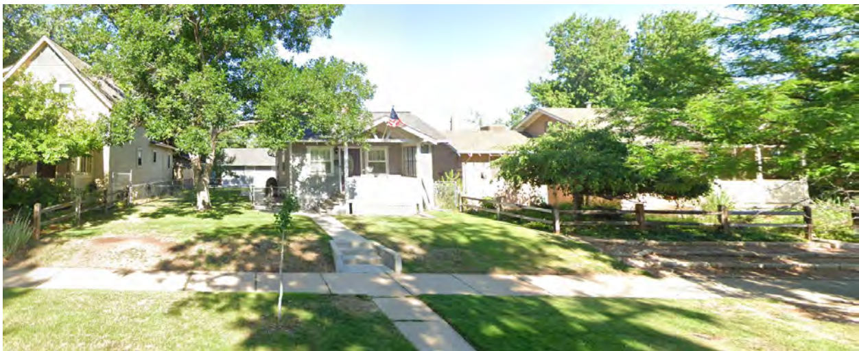
1825 S Marion St. - View of the subject property, looking west from South Marion St.
