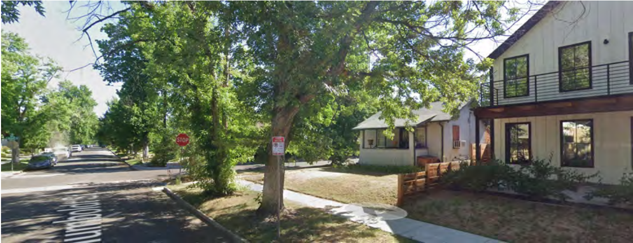
1900 S Humboldt St. - View of subject property, looking northeast from South Humboldt St.
