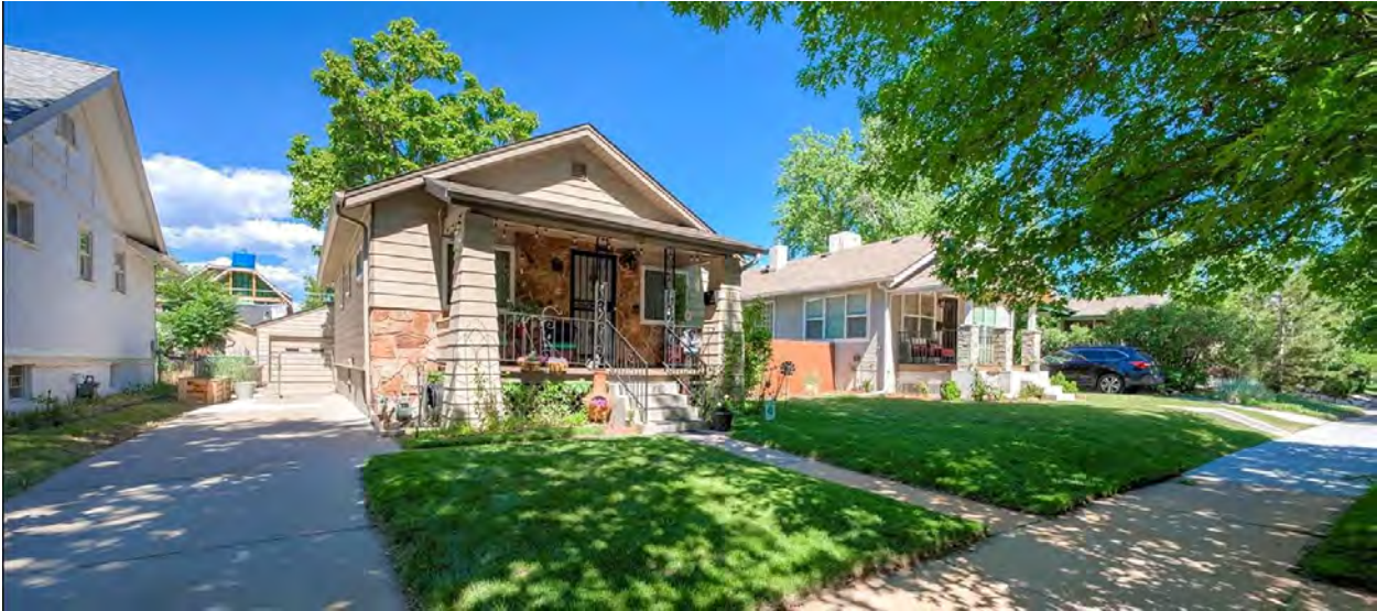
1931 S Humboldt St. - View of subject property, looking west on South Humboldt St.
