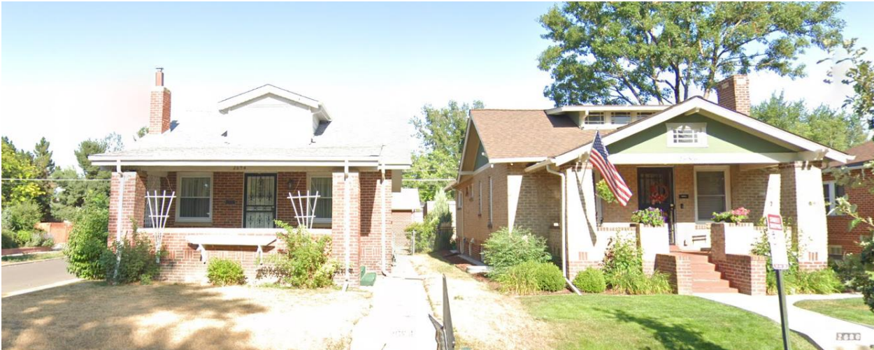
View of single family homes across the street of the Dahlia property, looking east.
