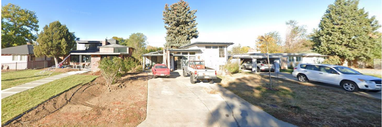
View of the Glencoe property, looking west.
