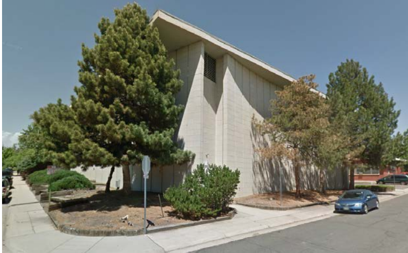
Northwest corner of Conejos Place and Stuart Street, viewing existing sanctuary on the subject site.
