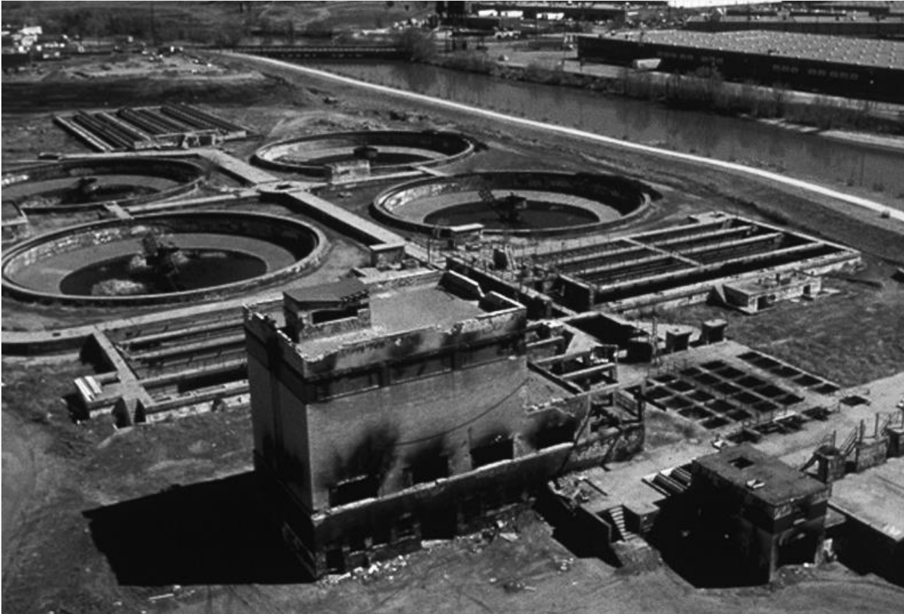
Northside Wastewater Sewage Treatment Facility
