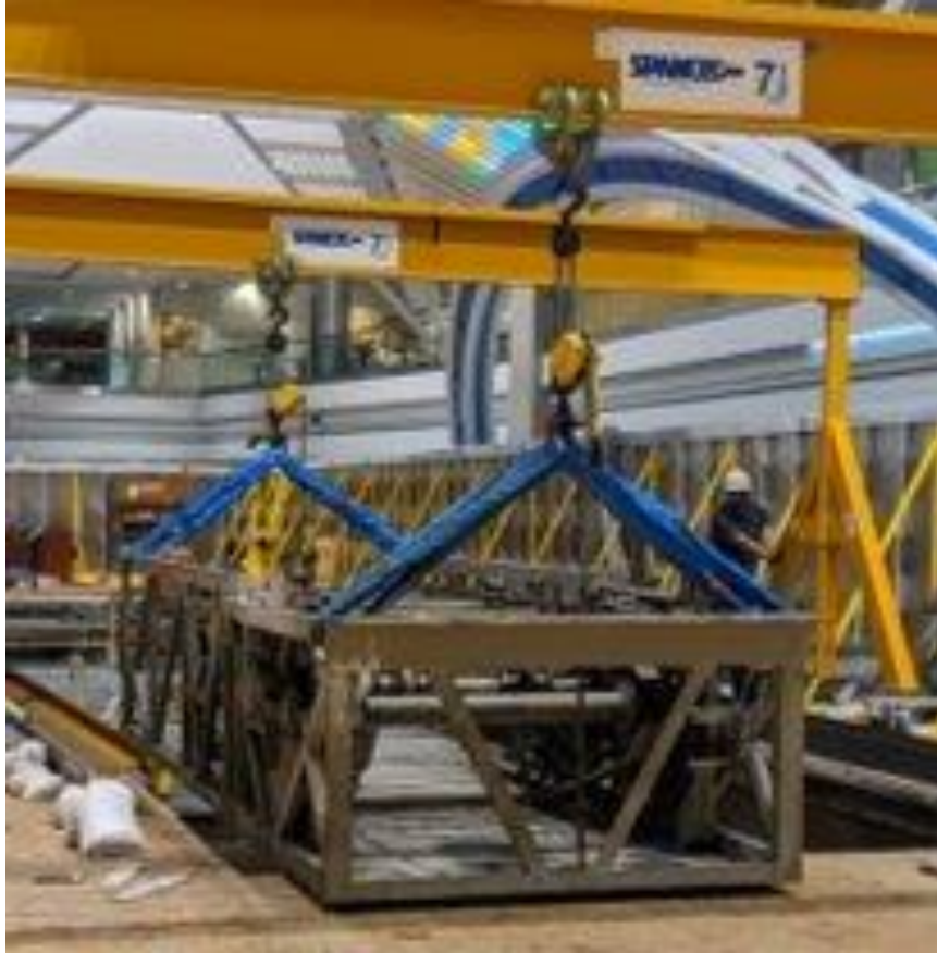
Removing Old Walkway
