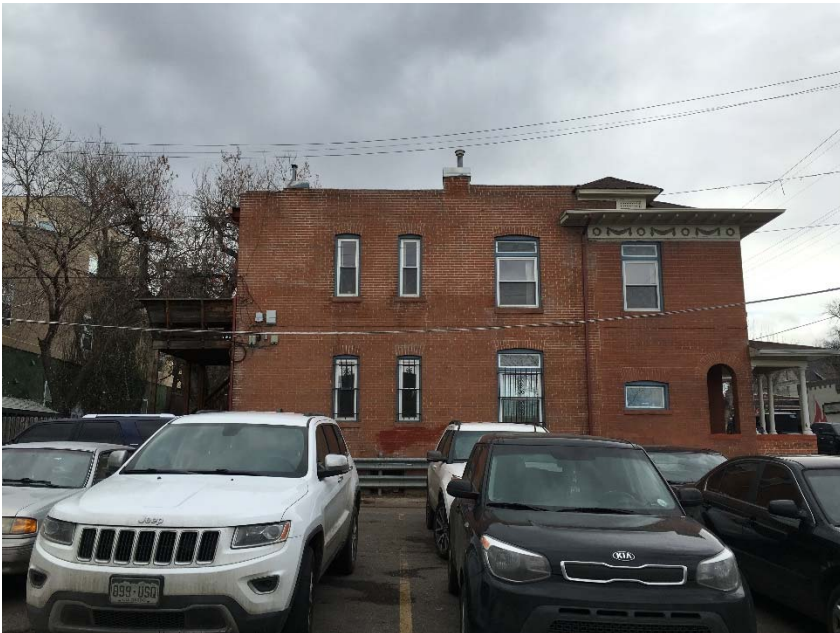
East Elevation of the Cole Apartment Building
