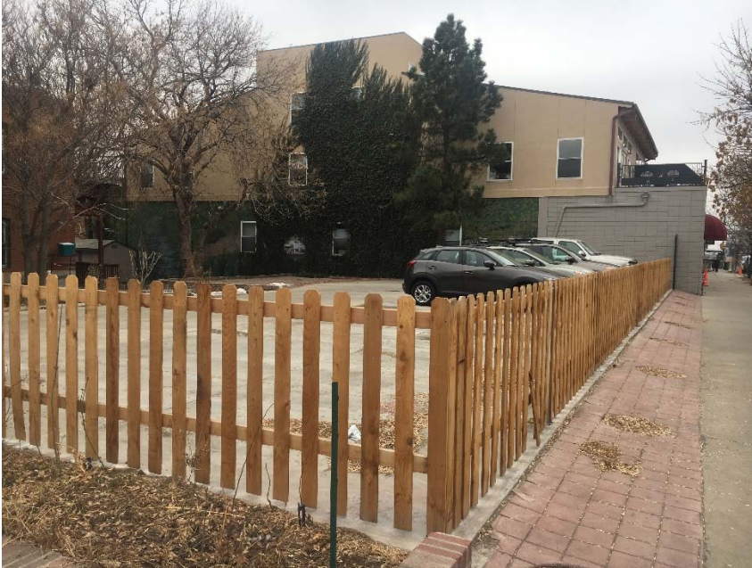
Northwest Corner Elevation
