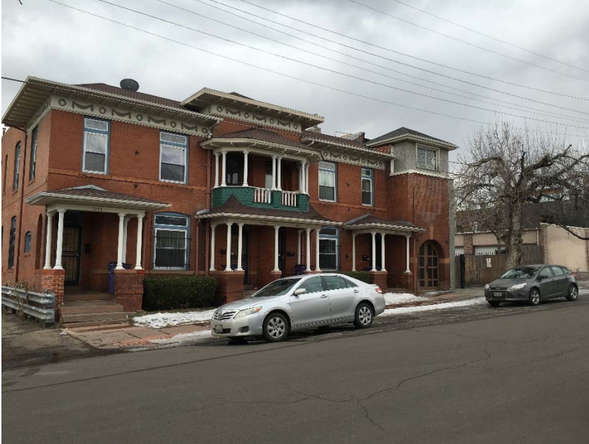
North Elevation of the Cole Apartment Building
