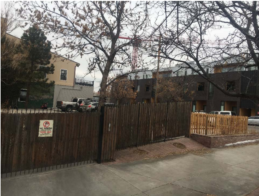
Northeast Corner Elevation
