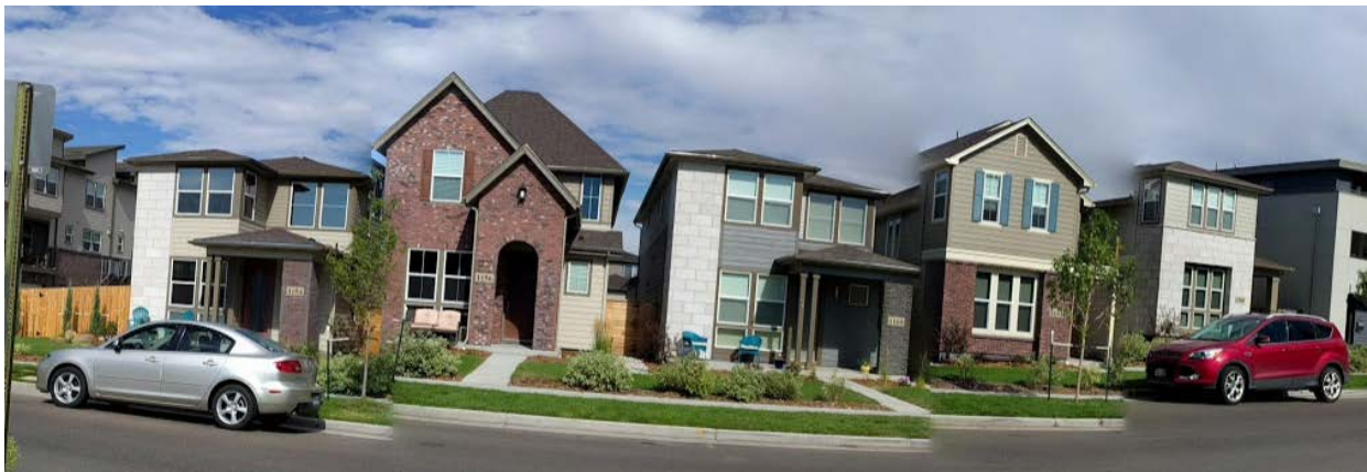
Subject site looking east.
