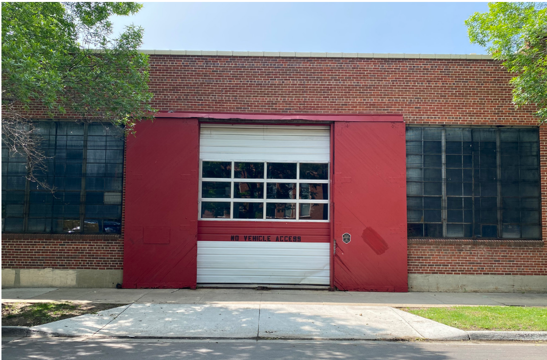
Figure 1-5 Existing North elevation showing historic windows, fenestration pattern, sliding barn doors, and solid to void ratio. Not to Scale. Illustrative Only.
