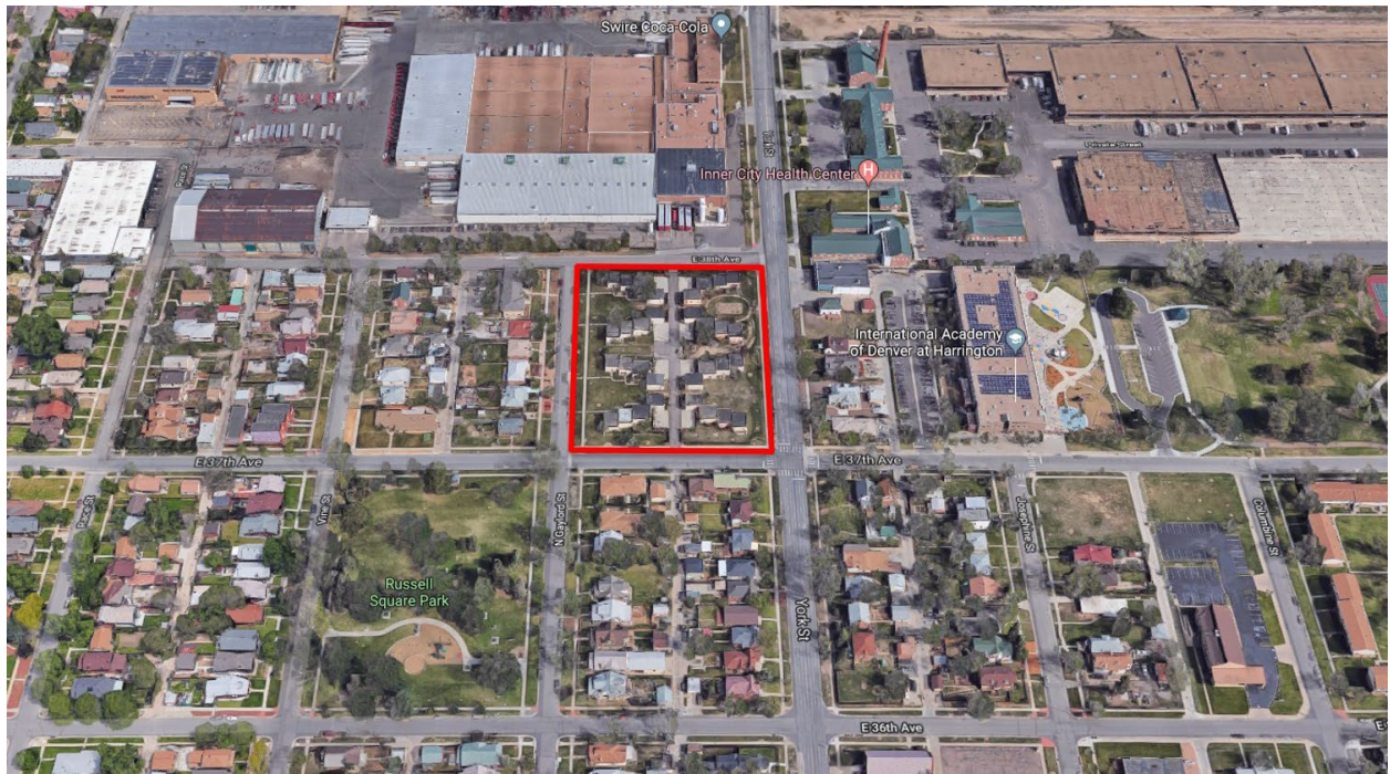
Aerial view of subject property, looking north.
