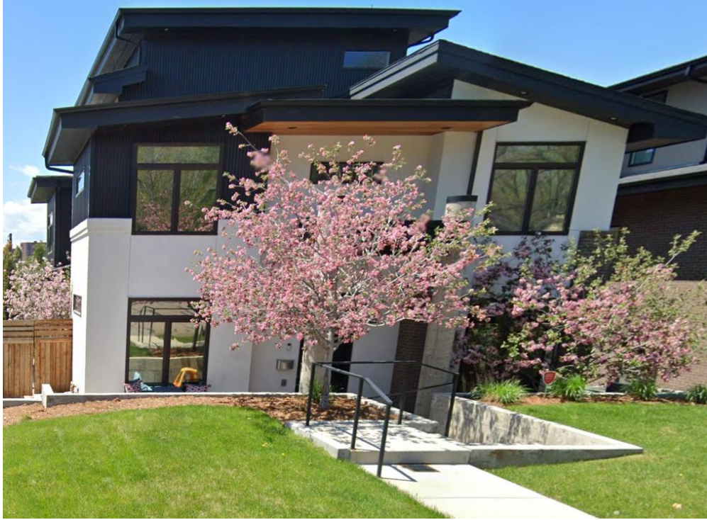
View of the property to the south, facing west.
