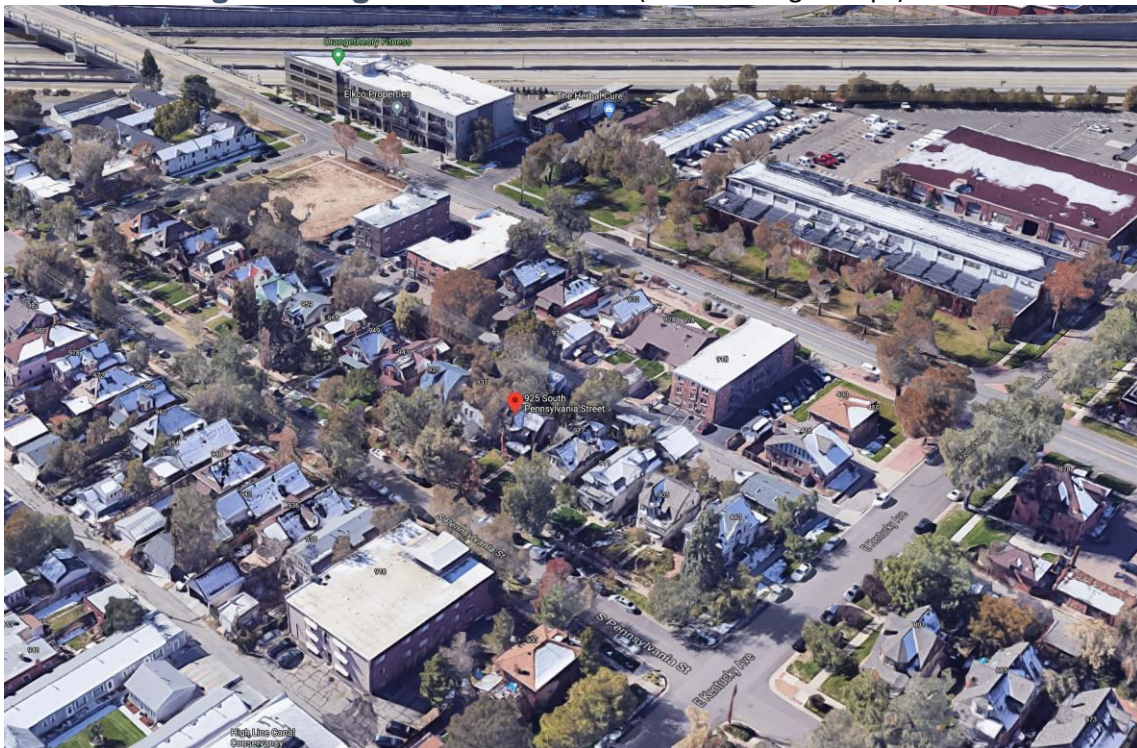
Aerial view of the site looking southwest.
