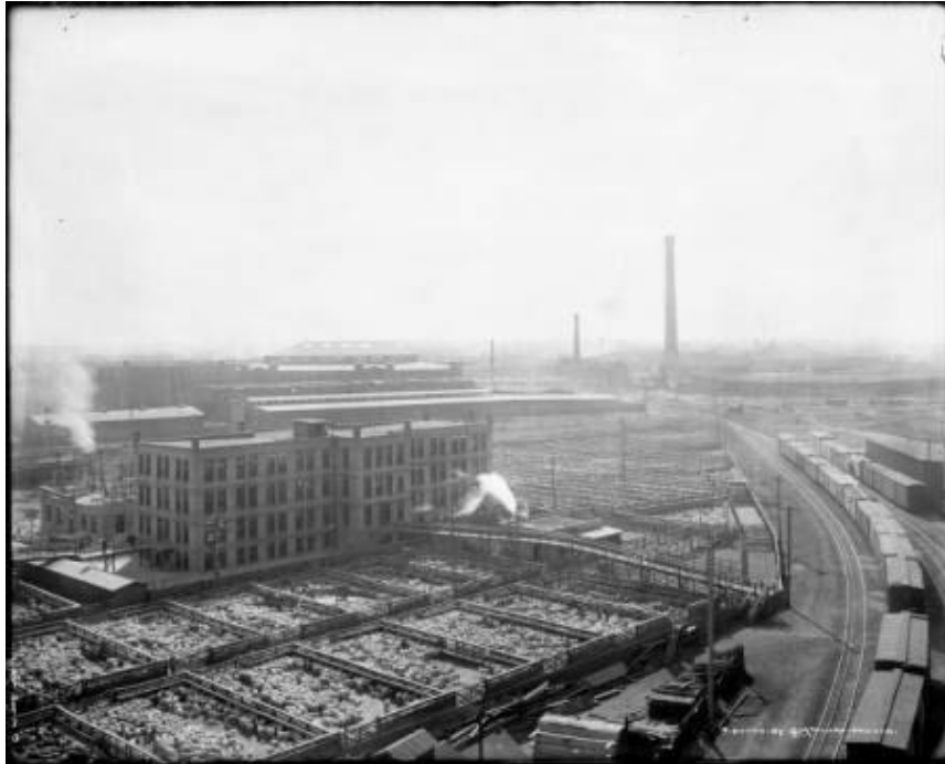
Figure 15. 1915 photo showing a train moving through the yards behind the 1898 structure. The 1916 structure is seen under construction. 71
