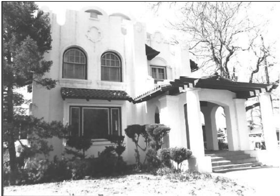
1899 York Street - Ghost/Rose House, West Elevation Photographed by Phyllis Smith, 1973 History Colorado Architectural Inventory Form, 5DV.2721
