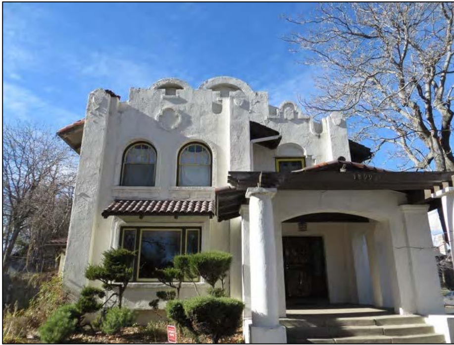
1899 York Street - Ghost/Rose House, West Elevation Photographed by Mason Seymore, 2016
