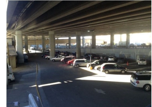
Under I-70/46 th Avenue
