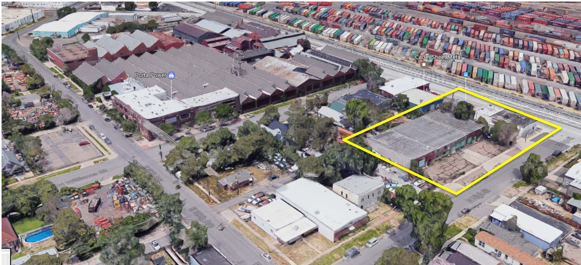
Aerial, looking northwest (Google Maps)
