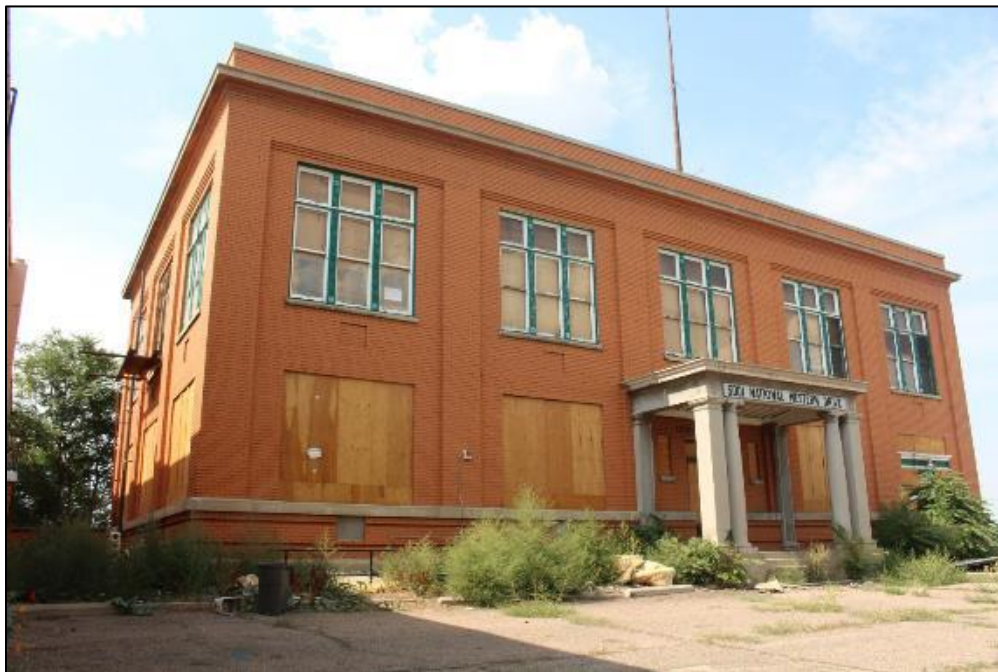
Armour Administration Building, front and side elevations, 2018
