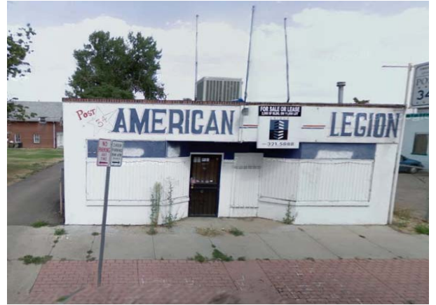
The property north on Tejon Street.
