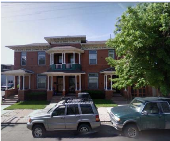
The property south cross 33 d Avenue.
