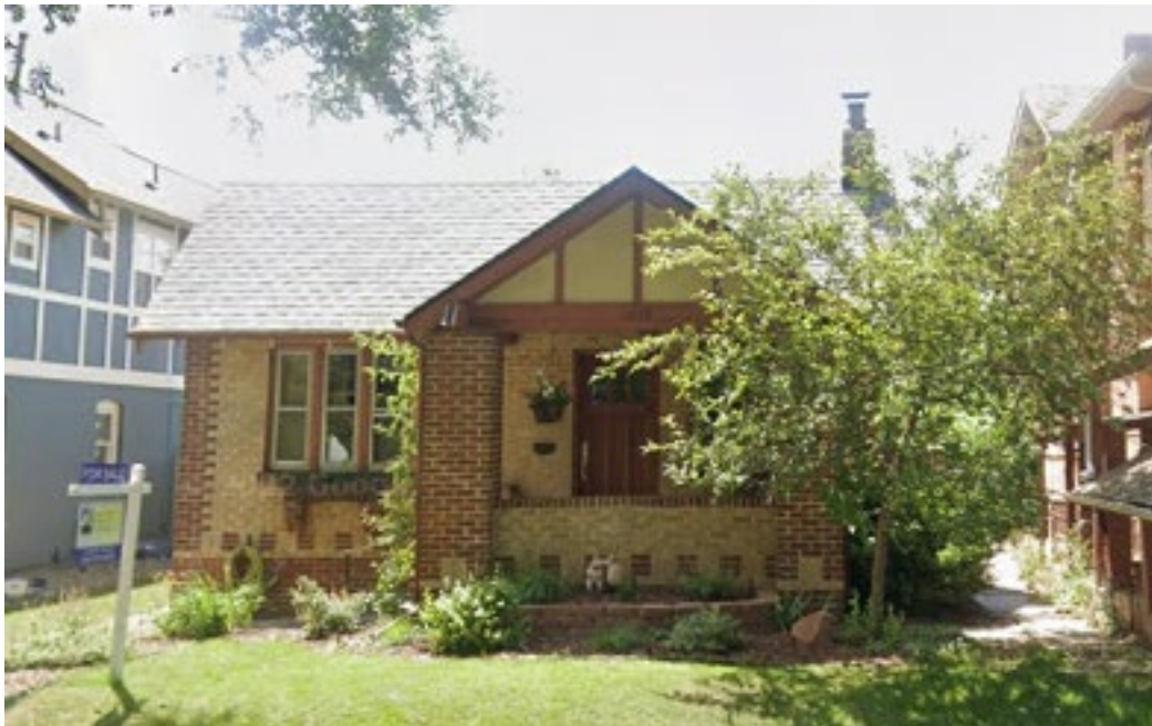
View of the subject property, facing east.
