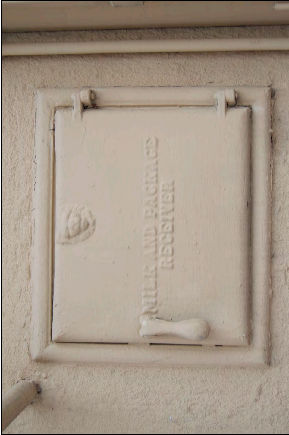
Door for milk and package delivery on the rear of 119 E. Vassar Ave.
