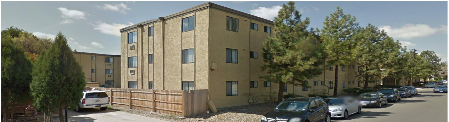
Subject site, looking southwest along Arkansas (Google Maps)
