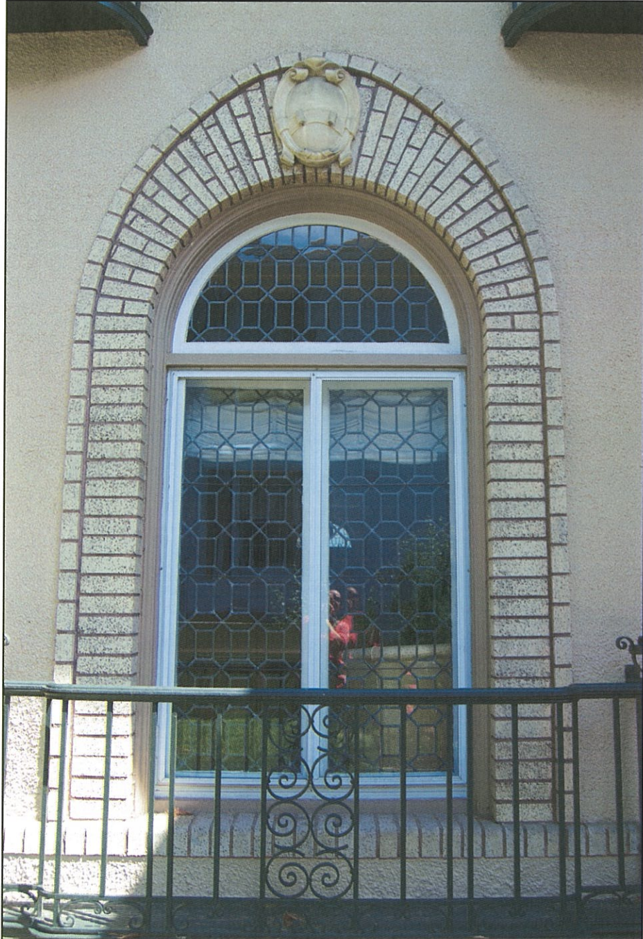
Window and details on south elevation
