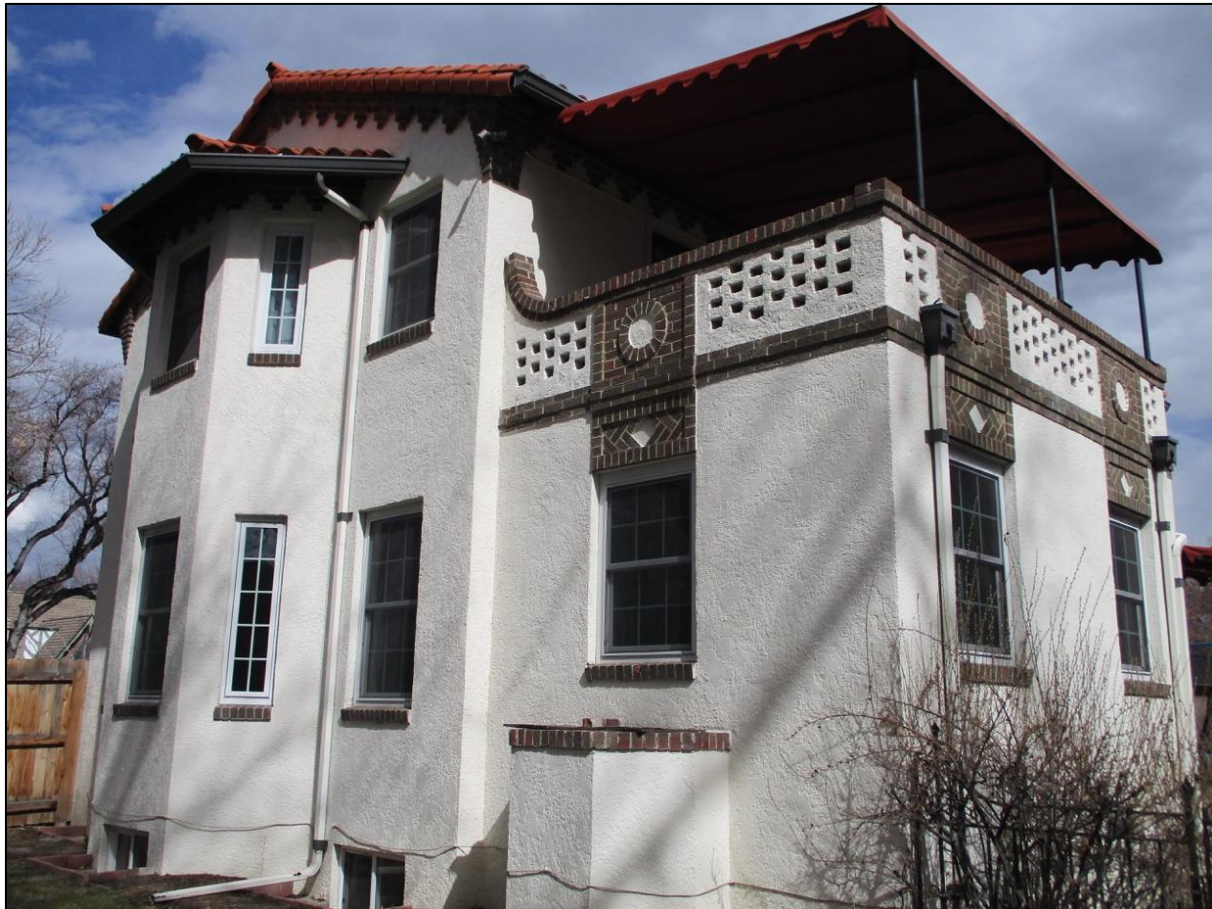
Figure 2 Looking northwest at side and rear elevations
