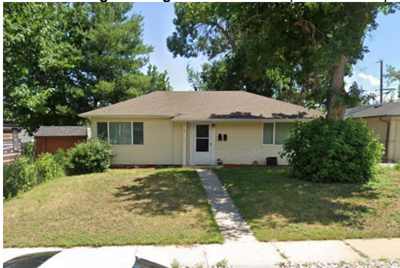
View of subject property looking east.
