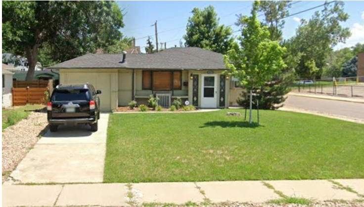
View of the property to the south, looking east.
