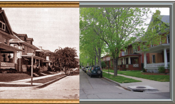
Frank S. Snell Subdivision Historic District. Historic photo on left 1911; current photo on right 2014.
