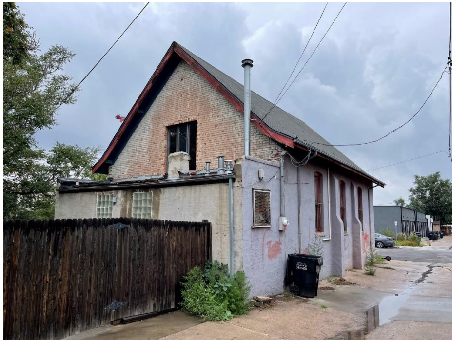
South Facade of 1618 E. 38 th Ave.
