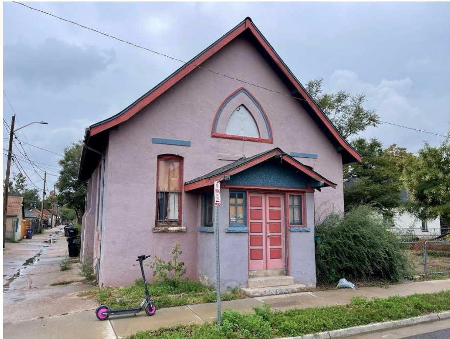
North Facade of 1618 E. 38 th Ave.
